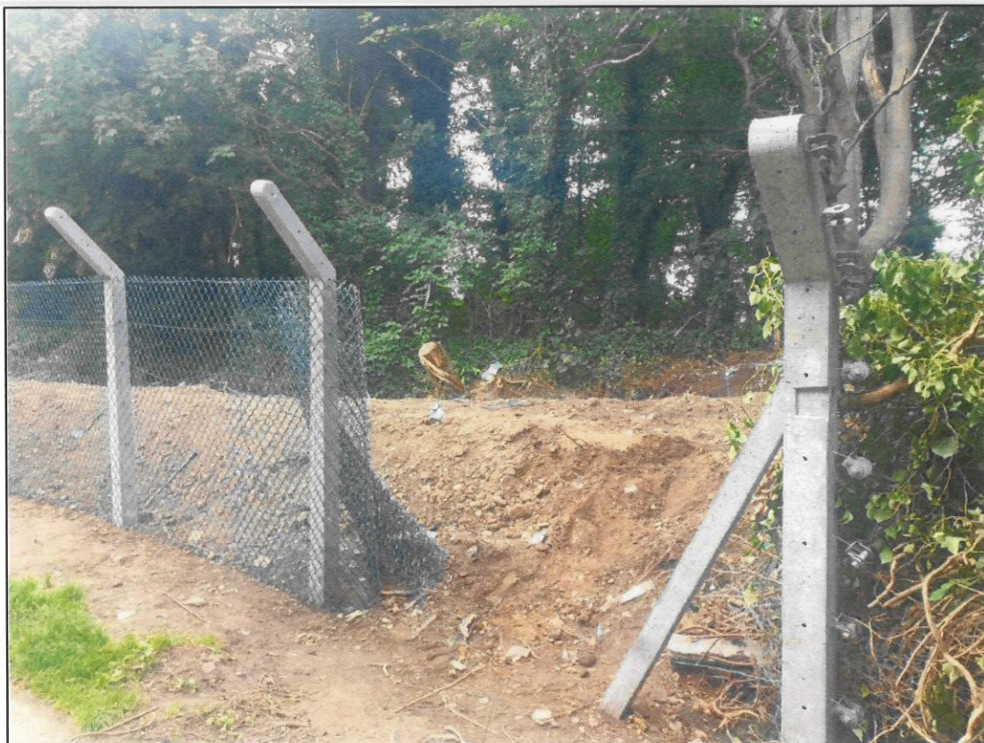
Figure 3: Fence Improvement and Maintenance Works
