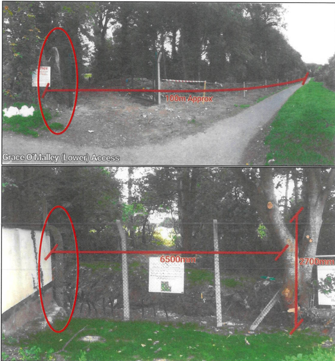
Figure 4: Photos from FIE Referral which illustrate existing 1970's fence posts (Annotated by TPA)
